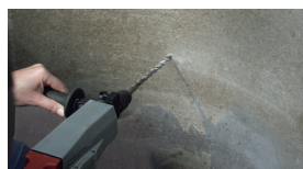
Easy installation - quick and reliable embedment: 1. Drill hole.
