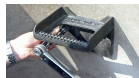
6. Position step iron anchor and tighten with a torque wrench with T_{inst} = 25 \text{ Nm} .
